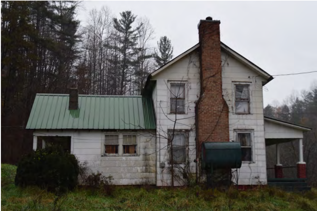
South gable end of the Caldwell House, view to the northeast
