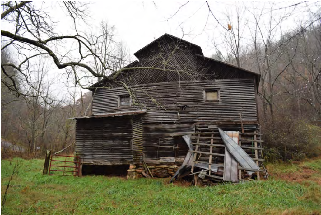
Livestock barn, view to the northwest
