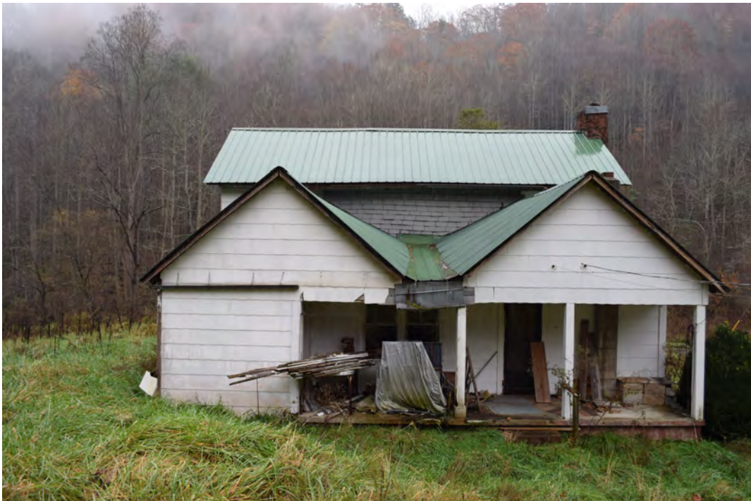
Rear elevation, view to the southeast
