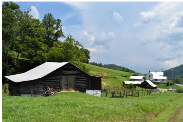
Outbuildings at the Clark Farm, view to the northeast
