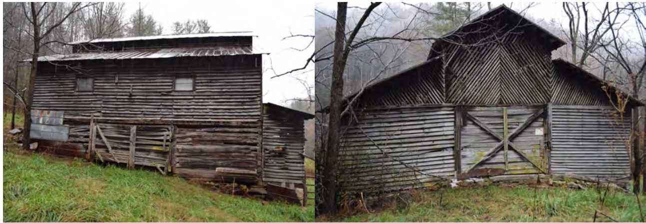
Livestock barn, southwest elevation (left) and northwest/rear elevation (right)
