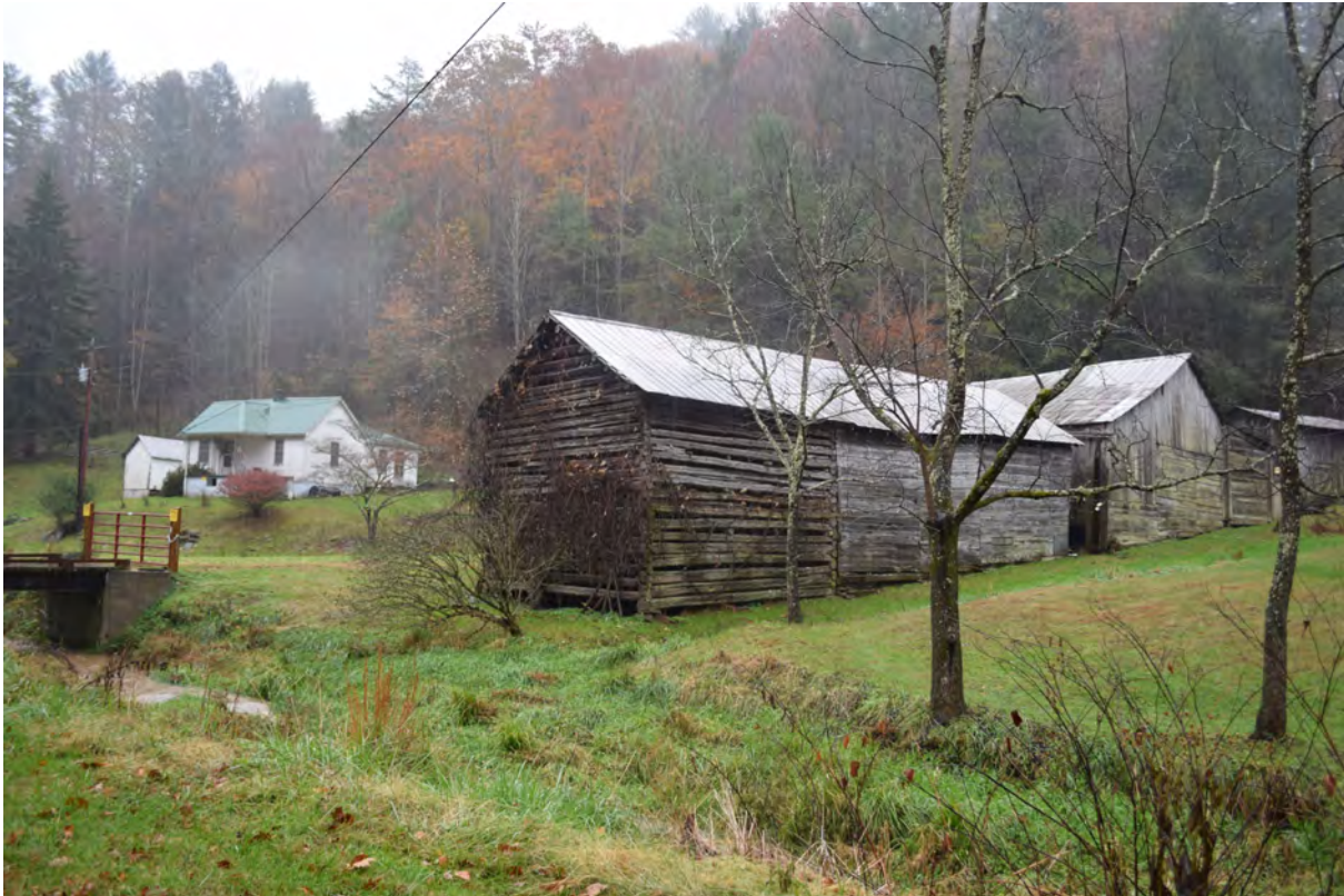
Plemmons Farm outbuildings with house in the background, view to the southeast
